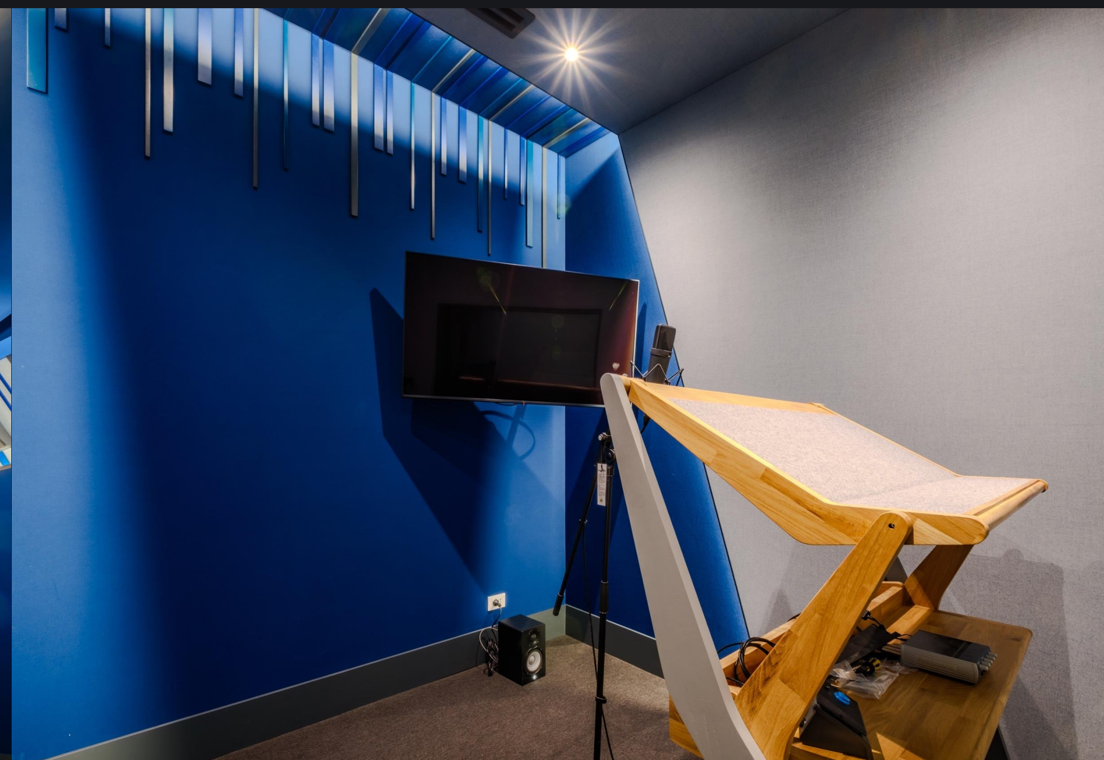
Booth detail: the slats are the treatment.
