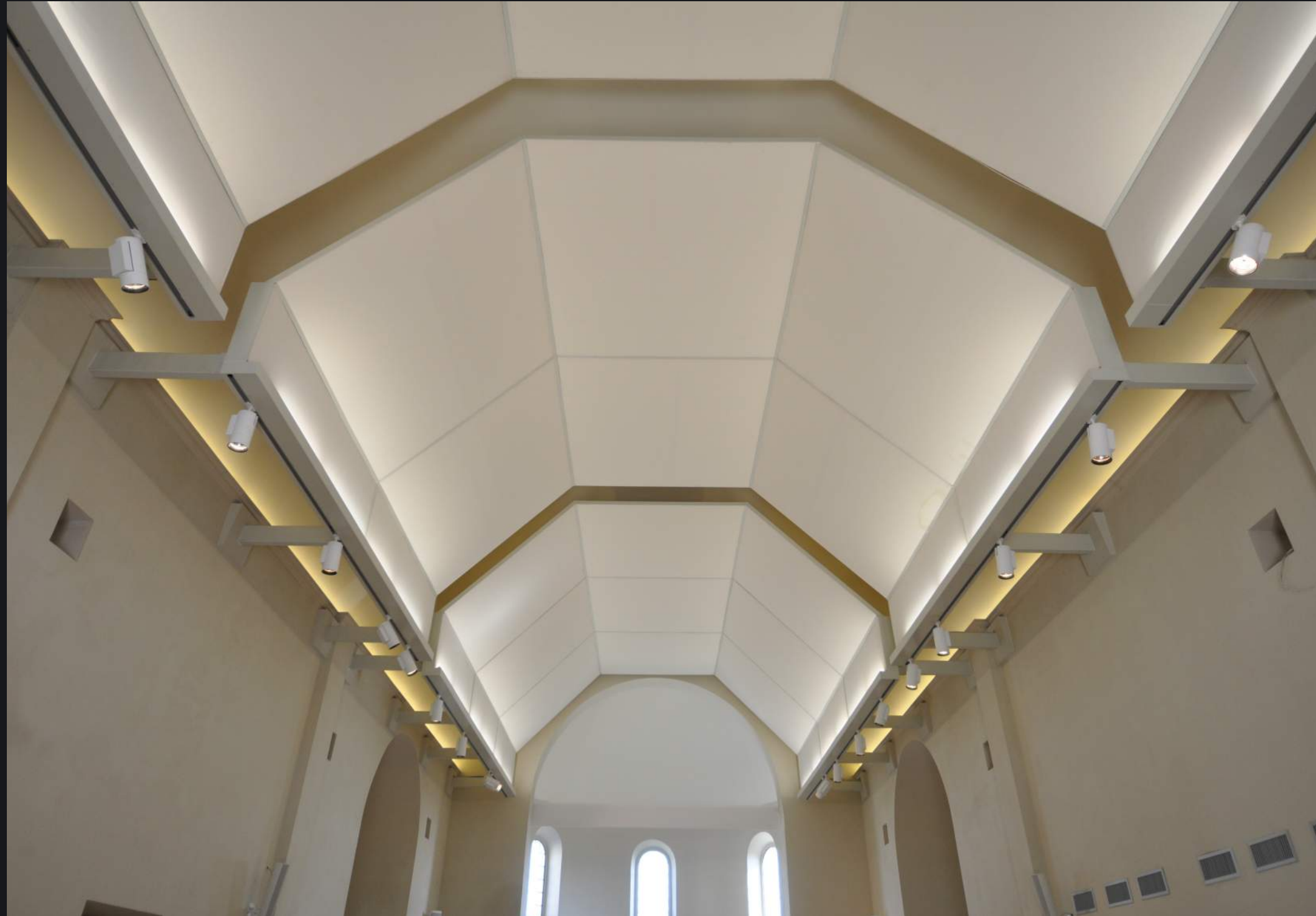
Acoustic Absorption with stretched fabric on the ceiling
